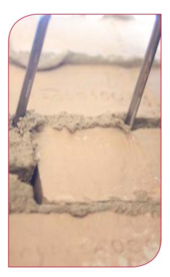
Placement and fixation of the anchor is carried out prior to the execution of the structure.
